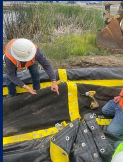
Figure 4. Assembling barrier panels on site
