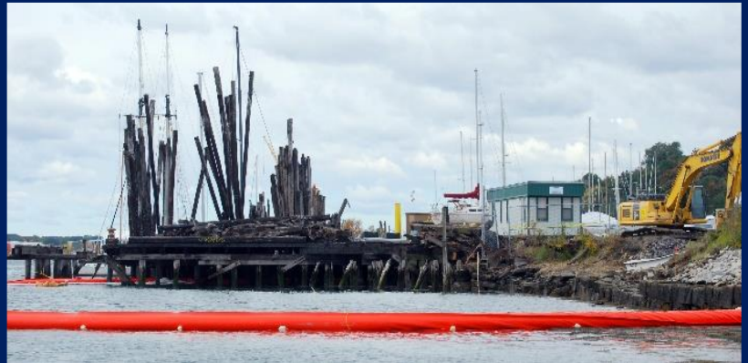
Figure 1. Portland Harbor, Maine. The system contains sediments, associated contaminants, and excludes fish and marine mammals, while allowing water passage.
